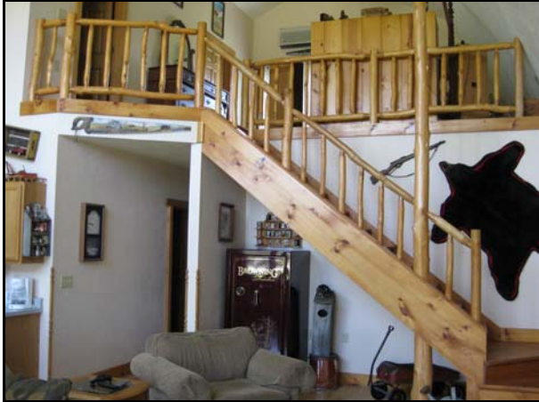
Loft—Aspen staircase, support & railing
